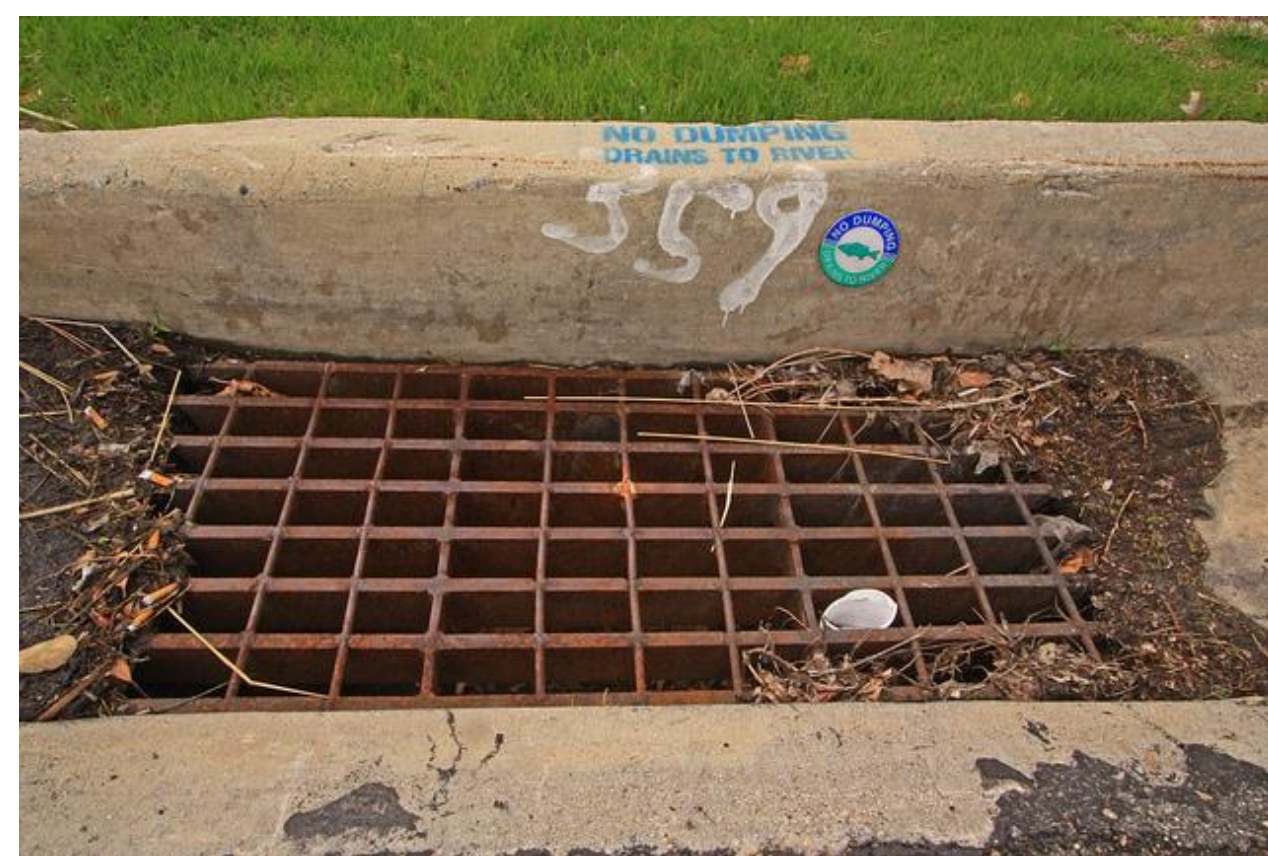
Figure 1. A storm drain in the Millcreek area of Salt Lake City.
