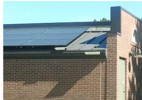
Figure 2: Assembled gutters to collect storm run-off from both solar panels and metal roof, USU Logan Campus.
