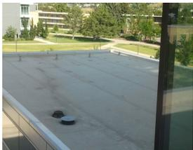
Figure 1. Flat membrane roof on ENG Building, USU-Logan Campus
