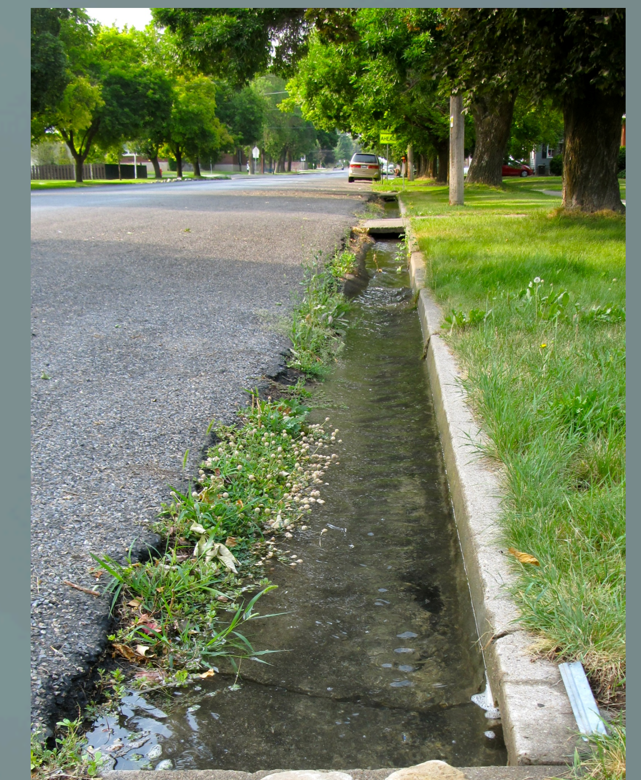
Figure 3. An example of overlapping irrigation and stormwater infrastructure
