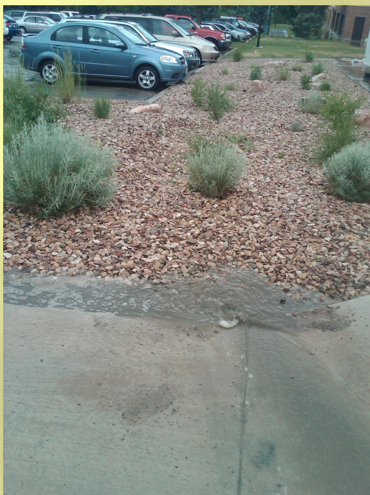
Figure 1. A demonstration bioinfiltration garden treating stormwater runoff from a driveway on the University of Utah campus during a spring rain storm.
