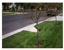
Cities across the West are exploring alternative stormwater management solutions. In Logan, Utah, a 'curb cut' is used to divert stormwater onto a grassy area. The water moves through the root zone and eventually into groundwater.
