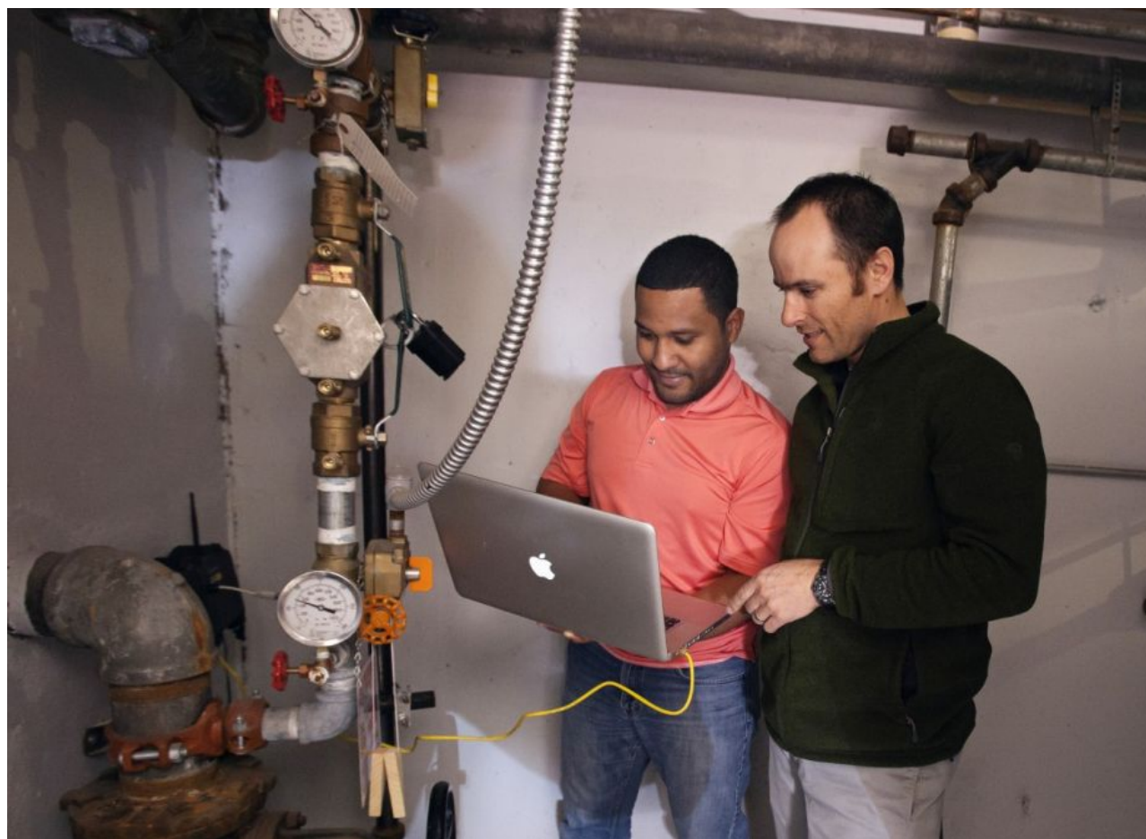
Jeff Horsburgh and graduate student Miguel Leonardo Feliz work to configure a smart water meter at a campus dormitory building. (Credit: Utah State University)
