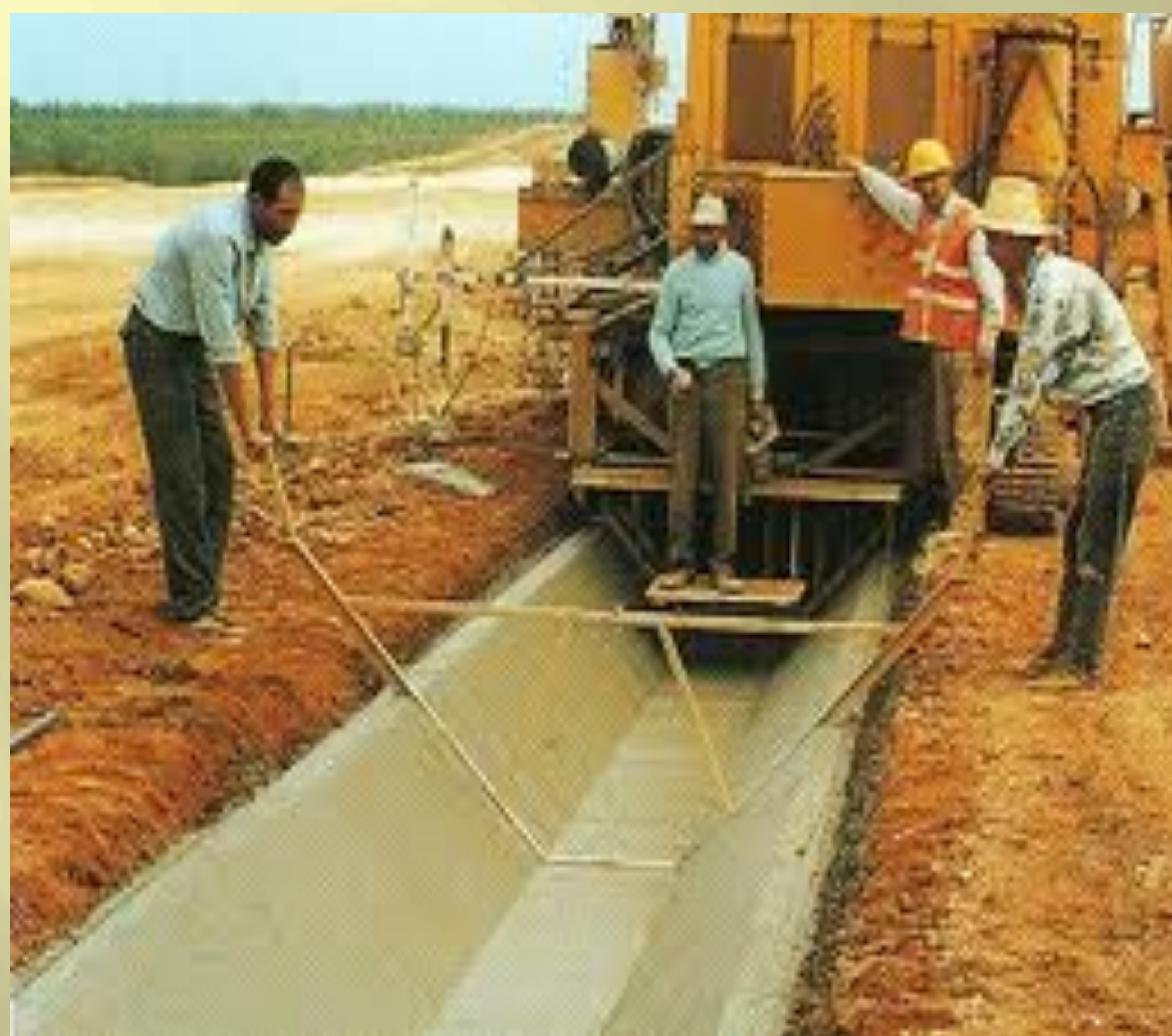
Figure 1: Canal Lining to mitigate seepage losses
