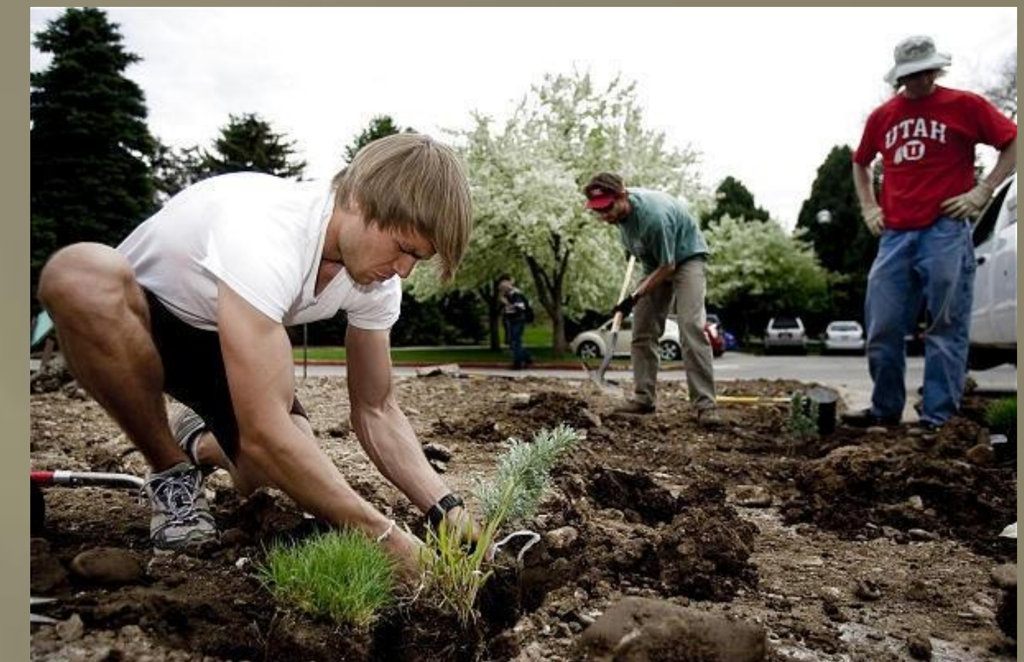
Figure 3. Thomas Walsh, Dasch Houdeshel, and Dr. Steve Burian building on-campus stormwater management practices.
